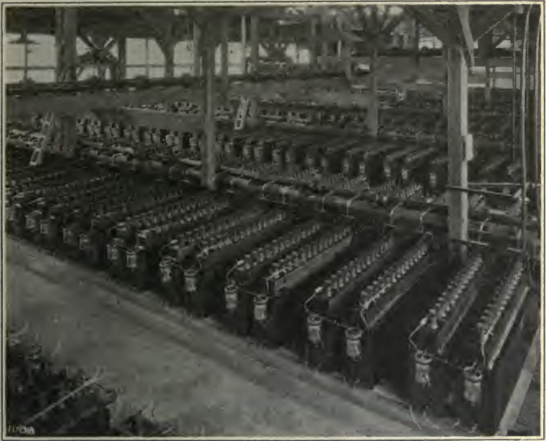
FIG. 21.—Interior View of the Cell Building.
